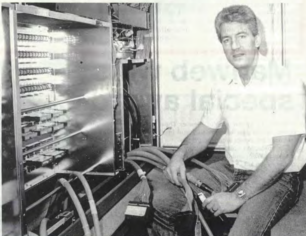
Computer Operations Manager Mike Gibbs lends a hand during the installation of the AMDAHL.
