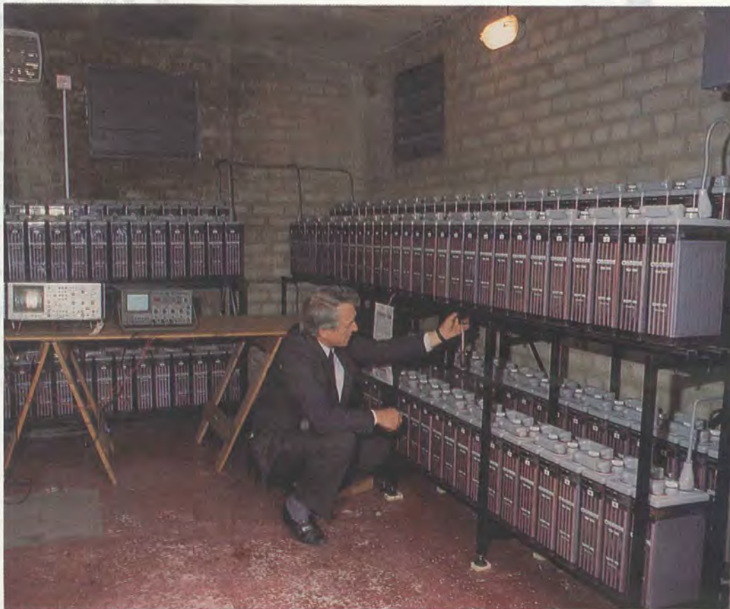
Eric Fisher is pictured checking the batteries in Box Lane Substation.
